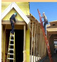
They are improperly using the top rung of this step ladder to work from.
