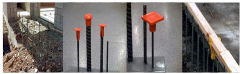
These rebar should be bent over or protected with caps so that a worker would not be injured by falling on
