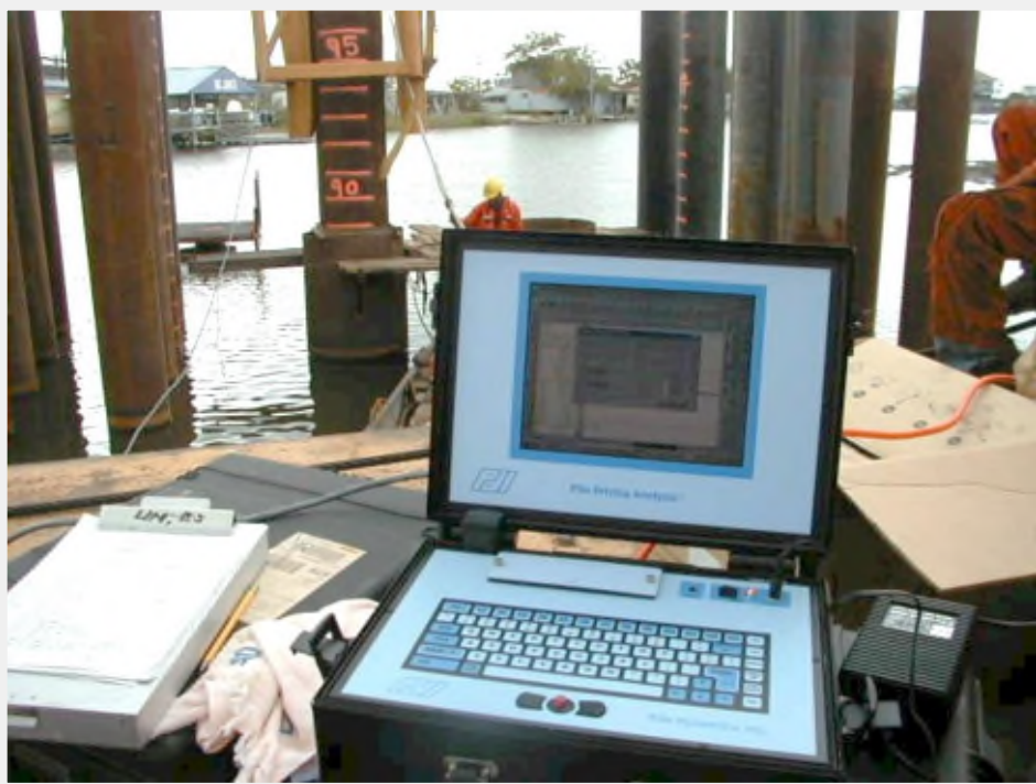
Preparing for PDA Monitoring
