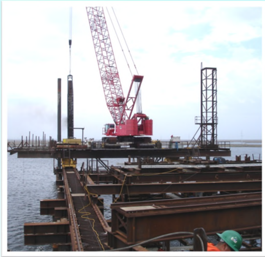
Lead Crane Driving Temporary Piles
