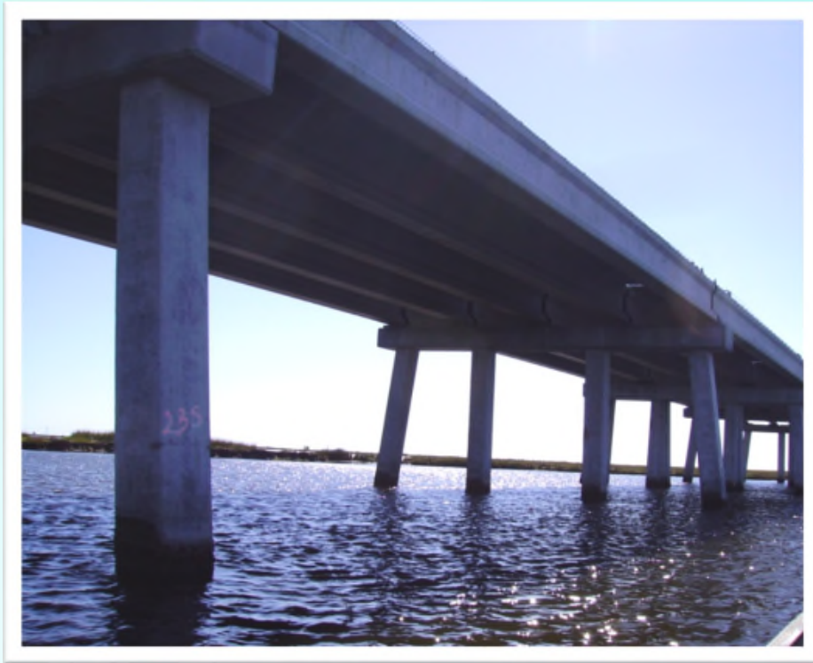
Elevated Highway on Phase 1
