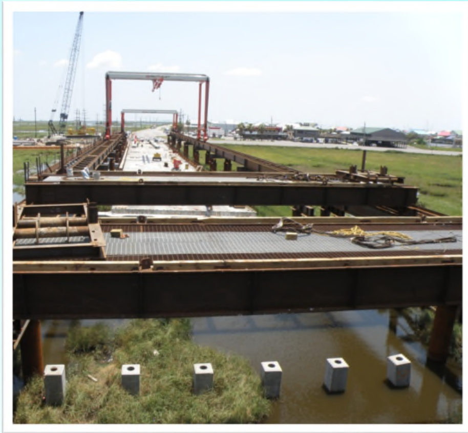
Permanent Piles Beneath Trestle
