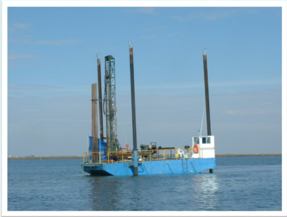
Drilling from Barge in Deeper Water
