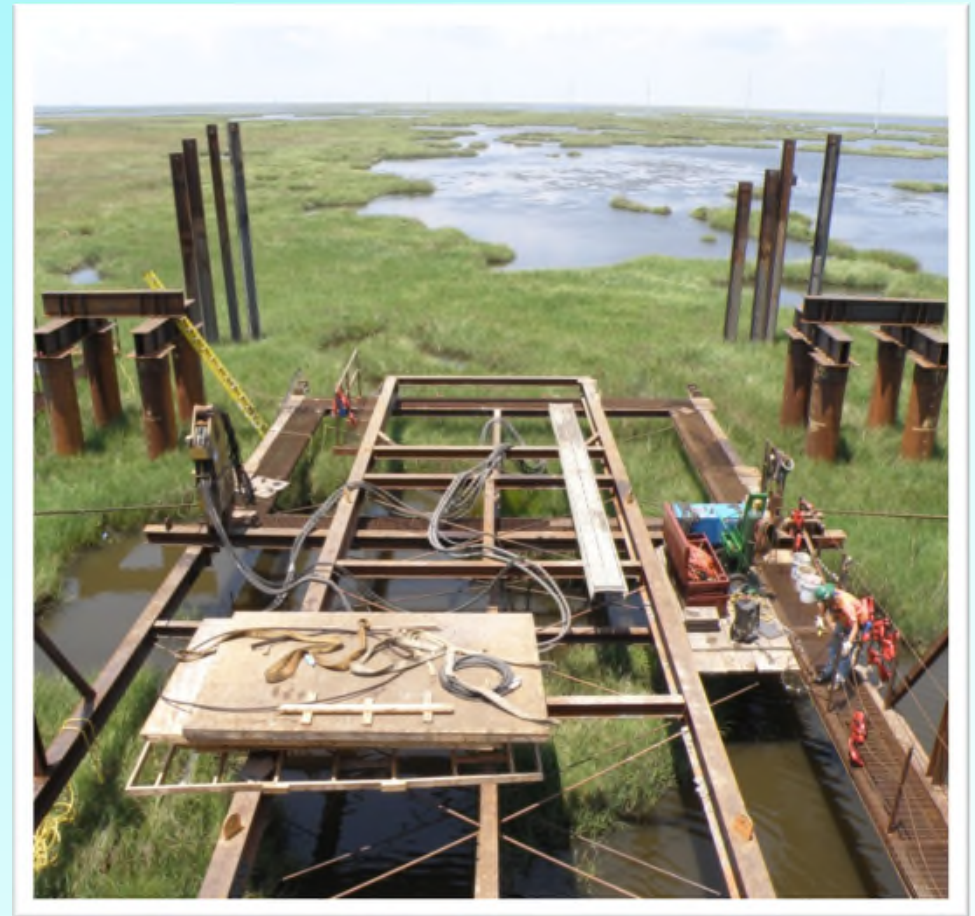
Looking off the Front of the Trestle
