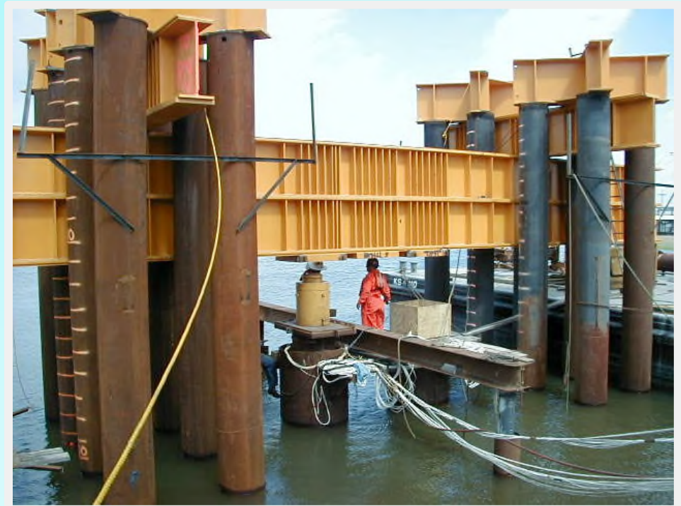
Static Load Test in Progress
