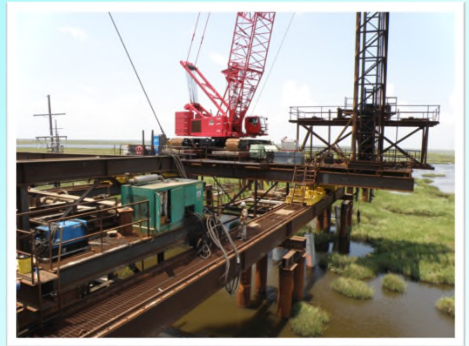
Pile Driving Crane and Hammer
