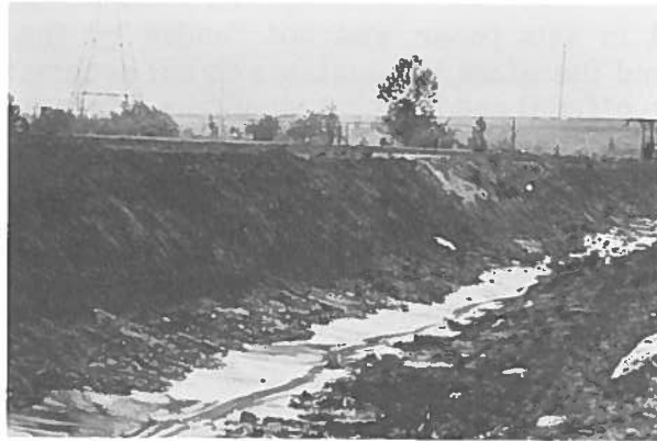
Figure 23. Completed Cast Gypsum Fly Ash Perimeter Dike.
