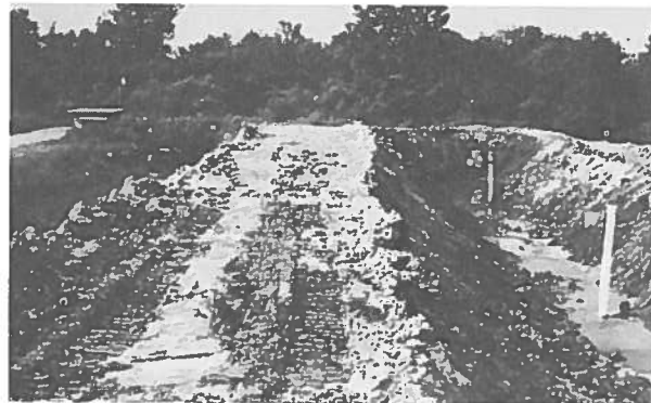
Figure 24. Completed Cast Gypsum Fly Ash Perimeter Dike.
