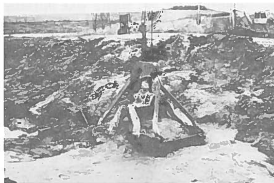
Figure 22. Casting of "Wet" Gypsum Fly Ash Waste.
